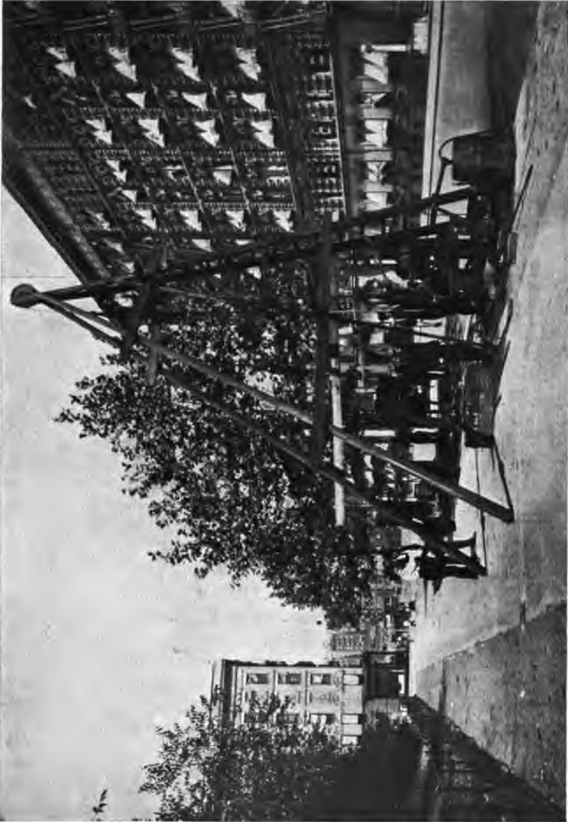
PLATE 20.—Sullivan Hydraulic Diamond Drill in New York City. Steam furnished by portable boiler and rods raised and lowered by tripod derricks operated from drum of drill.
